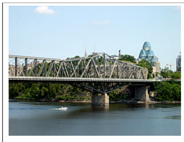
Exhibit 2 - Alexandra Bridge from Ottawa, Ontario to Gatineau, Quebec
