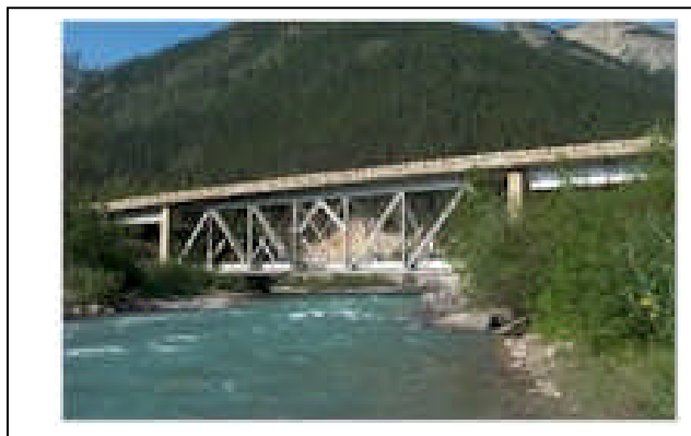
Exhibit 5 - Trout River Bridge, Alaska Highway, British Columbia
