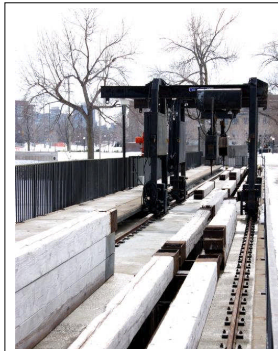
Exhibit 4 - Rideau Falls Dam Ottawa, Ontario
